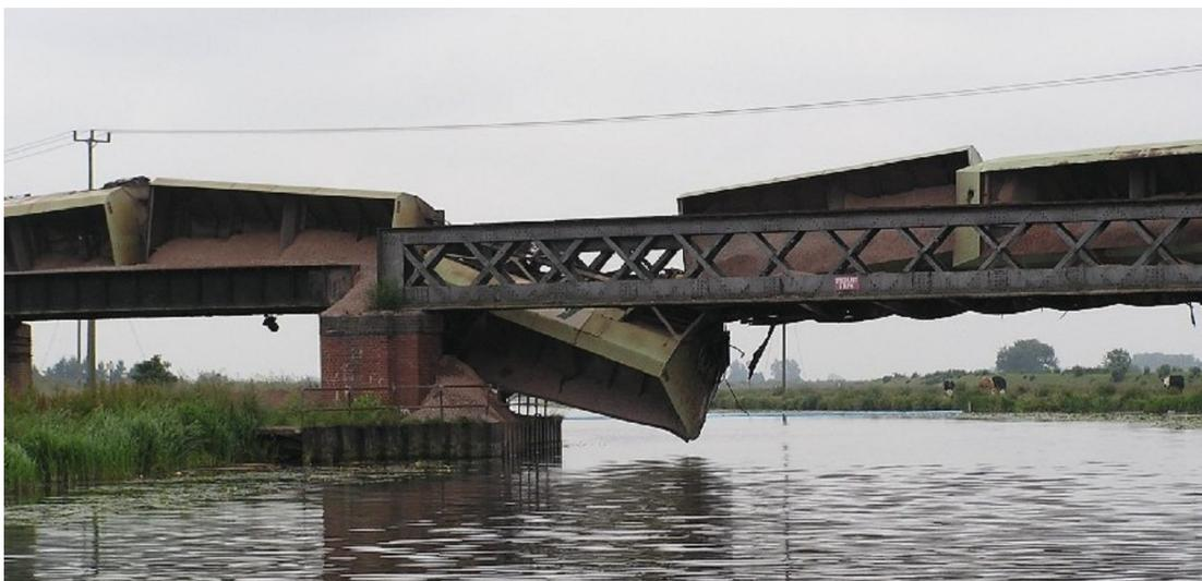
The nearest road was about half a mile away across very marshy ground and the only option was for Network Rail to construct a track to enable a heavy duty crane to be brought to lift the wagons off the bridge. It took two weeks to carry out site
