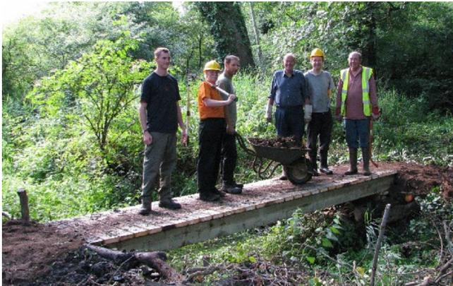
woodland end and then the first tread board. Meanwhile the course of the new footpath back to Weavers Way was cleared and improvements made to the existing section of the path. The bridge was completed in the afternoon with wire netting being laid and stapled onto its surface and the approaches being earthed up. The final task was to test the new structure, and it passed with flying colours.
