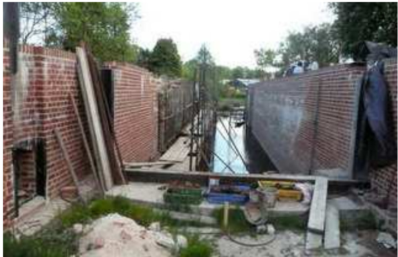
Right: Bacton Wood Lock showing the right hand wall that has been completely re-built whilst part of the left hand wall has been similarly re-built with scaffolding up for work to be completed on the remainder.
