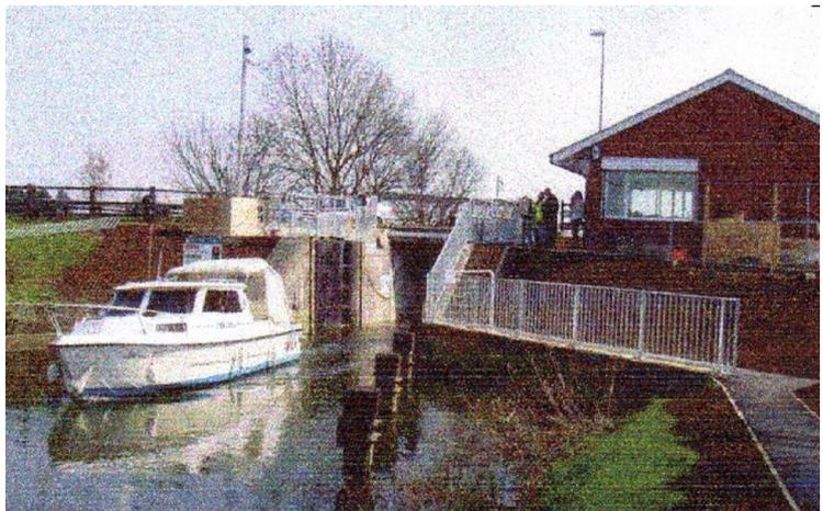
The work has not come cheap. Over £350,000 alone has been spent on installing new power packs, cables, actuators and electronic control panels replacing the old obsolete system. The new building is four times larger than the old and besides housing the lock controls has an information room and toilets and showers for boaters to use. New traffic lights have been installed to control the passage of boats through the lock. Our picture shows a cruiser leaving the lock on the re-opening day.
