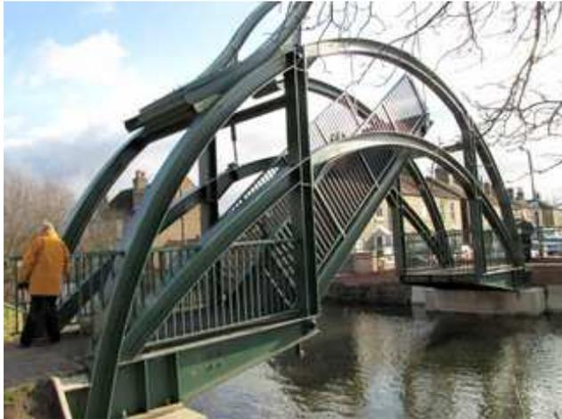
At the same time the new hydraulically-operated lifting bridge will also be formally opened. Although largely installed at the end of last year some modifications were needed to ensure it operated properly and these snags had been sorted out by the end of March enabling it to be operated more easily. This all reflects great credit on the SNT.
