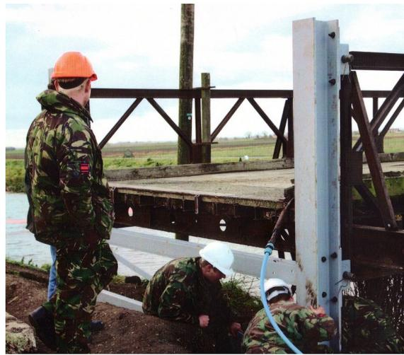
Two more pictures of the splendid work on the Ramsey Hollow Bridge over the Forty Foot River. On the left the old bridge has been jacked up on temporary timber supports (and is that a narrow boat waiting to pass under?). Whilst on the right one of the new steel uprights is now in place and is being fixed. We are grateful to Nigel Long and Jim Shead of IWA Peterborough Branch for these two pictures and that on page 7 of the finished bridge.
