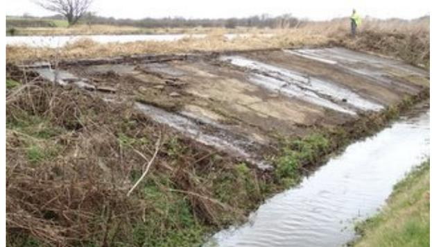
A major objective was achieved on 23 February when the overgrown spillway, above Ebridge Lock, was cleared enabling it to be able to function by allowing surplus water to flow into the back soke. Some repairs will eventually be needed but in the meantime this important flood protection measure is now fully functional.
