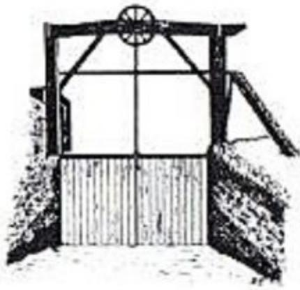
Guillotine staunches usually consisted of a shutter or clough raised vertically out of the water by chains. That at Bone Mill, on the Nar, (left) was raised by the operator climbing the ladder and turning an iron wheel to open the gate. On the Nene, there was a single roller, operated by crank handle, to raise the gate. However, on Bottisham Lode
