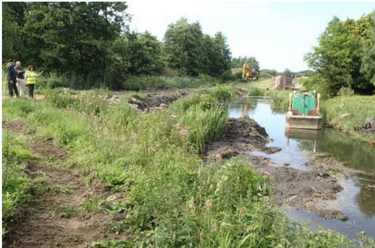
The third picture was taken on 30 August at Pigneys Wood and shows work in hand on moving a small footbridge over the soke dyke to allow machinery to access the canal there. It shows the large digger making light work of lifting the heavy bridge and re-positioning it.
