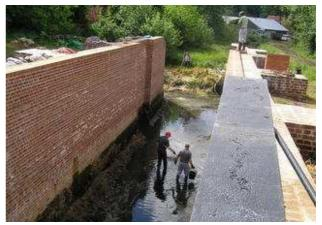
Inside Bacton Wood Lock before the chamber was finally drained down. Already there is a steep drop down from the top sill as shown on the left, whilst on the right the volunteers clear small fish from the chamber. (Alan Bertram)
