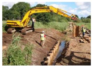
(Left) The start of the quay heading work alongside the site of the former Wherry Inn at Royston Bridge whilst (right) a short distance away work gets going on the complete rebuilding of the old spillway.
