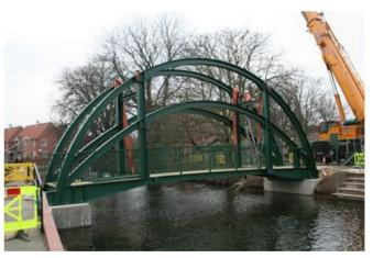
inserted. Centre Right: Parts for the new lifting footbridge at Sleaford were delivered from the Hucknall factory on two lorries on 29 December and had to be erected on site before the structure could be craned into position across the river. Bottom Right: The new structure is in position and nearly complete, apart from fitting the counter weight which is about to take place, and the installation of the lifting mechanism which followed on at a later date.
