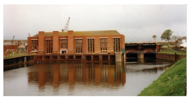
The Black Sluice pumping station at Boston. The London Road runs behind the station and the new entrance lock is to be constructed on the far side of that road with boats entering the new navigation through the existing passage on the right, where the top of the arch carrying the road is just visible.
