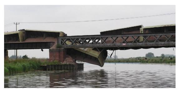
The nearest road was about half a mile away across very marshy ground and the only option was for Network Rail to construct a track to enable a heavy duty crane to be brought it to lift the wagons off the bridge. It took two weeks to carry out site
