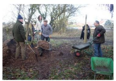
Honing Staithe Walk: 0n 12 January 2014 many barrow loads of chippings were laid on the path through the wood to consolidate the surface for walkers. When it was created the path had to be routed through low lying land that was liable to flood and building up its surface will make for a much firmer surface in future.
