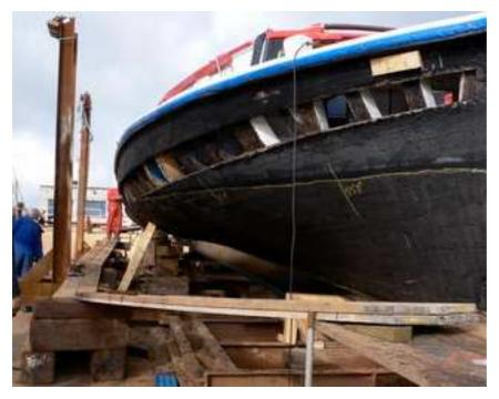
Once on the slip tar was scraped off the hull whilst the boatbuilders about set removing old the frames designated for removal on this occasion. As the tar was removed, armed with a drawing board and pencil I produced a schematic of the hull showing the location and length of all planks. This was followed by a condition report on each one ranging from "sound" "horrendous".
