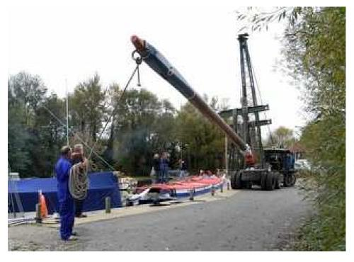
Whilst all this work was underway new mast was being roughed out at International Boatbuilding College within 200 yards where Albion lay on the slip. The Trust had obtained baulk in the mid-1990's and decided to have it worked up as a spare.
