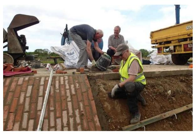
For the sessions in May and June work has been concentrated on facing the Royston Bridge spillway with brickwork – this having to be laid on a prepared surface at a 45% angle to the vertical. With the angle involved this turned out to be a relatively skilled operation but one the volunteers took in their stride with Laurie Ashton over-seeing progress.
